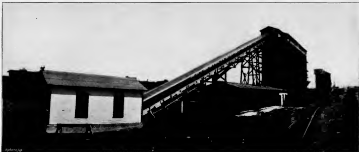
CENTRAL OF NEW JERSEY LOCOMOTIVE COALING PLANT—COAL WHARF AT ELIZABETHPORT, WITH ROBINS BELT CONVEYOR.
